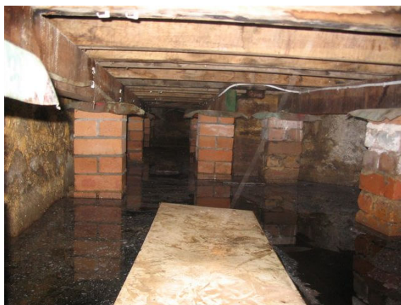
Figure 5.1: Existing seawater ingress below flooring system (approx 1.90m ISLW)
