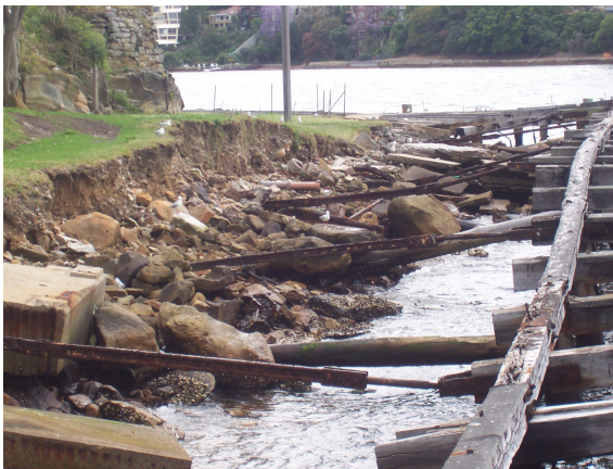
Figure 5.2: Foreshore recession and failed ad-hoc protection works in South Depot Precinct
